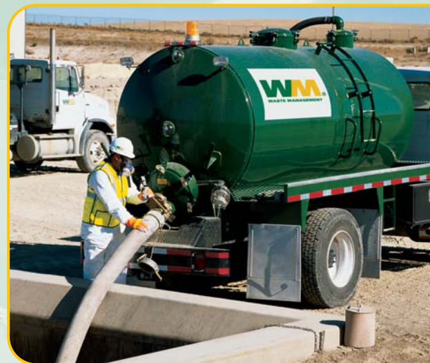
LiquiFix SM solidification begins with the pumping of liquid waste into a lined basin. Reagents and/or absorbents are then added to the mixture.
