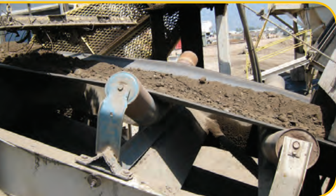
Discharged media is clean, contaminant-free, and ready for reuse.
