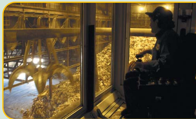
Wheelabrator facilities are specifically designed for the total destruction of large quantities of waste products, including confidential documents.
